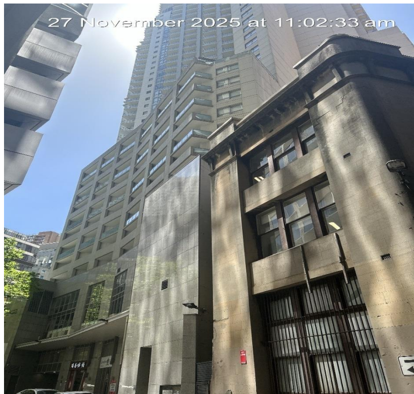
Figure 1: 2-4 Cunningham Street, Haymarket, viewed from the east
